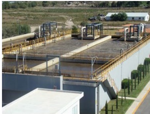
Reactor aerobio
