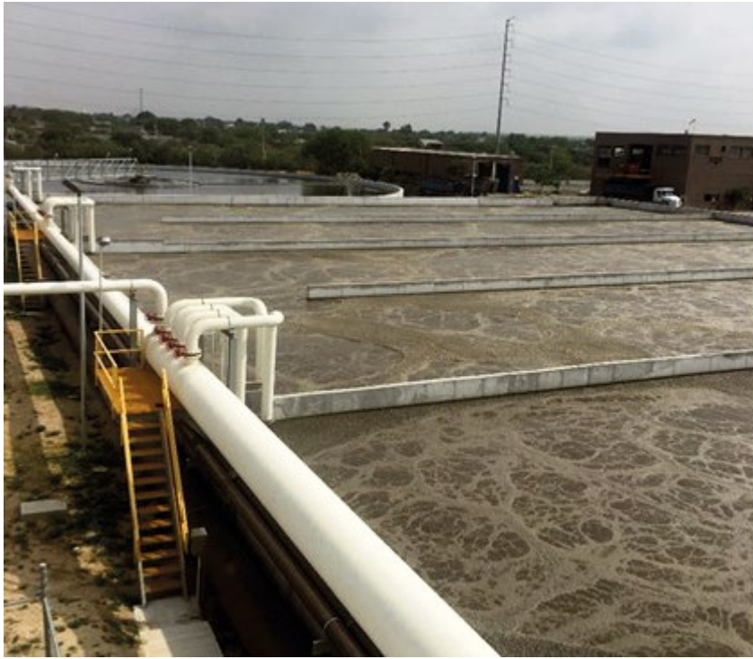
Reactor aerobio
