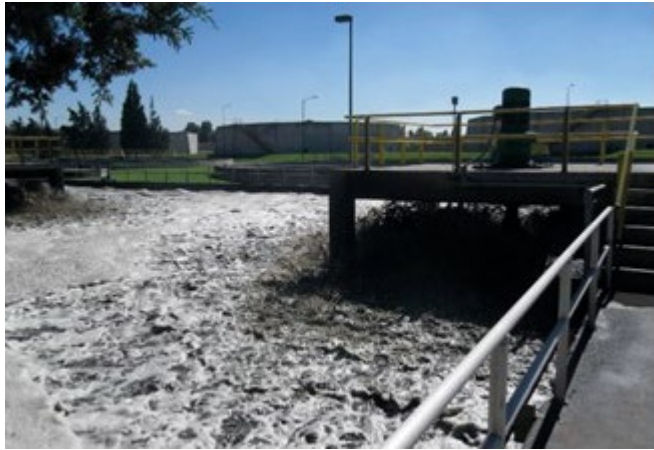
Reactor aerobio
