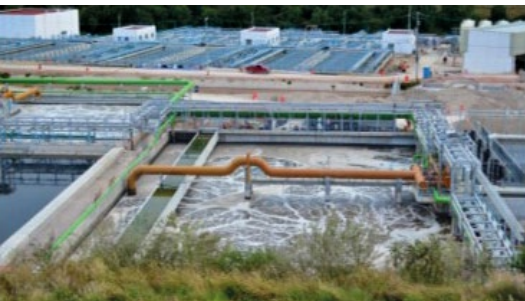
Reactor aerobio
