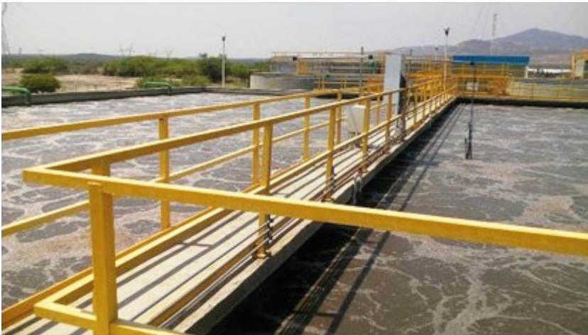
Reactor aerobio
