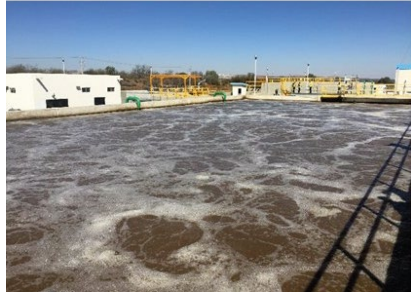
Reactor aerobio
